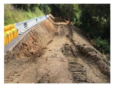
Excavation to continue for installation of gabion retaining walls at southern section, Chainage 6970
