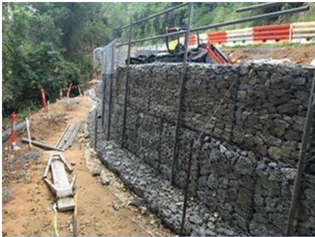
Gabion Wall G1 (looking south) towards bored piers area
