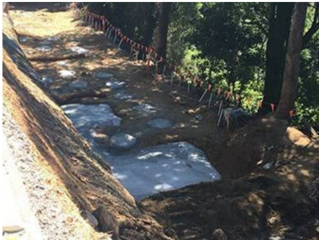
View looking north at CH 6700 showing concrete piers installed for Gabion Wall G1.
