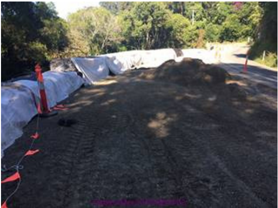
Progress with Wall G6
